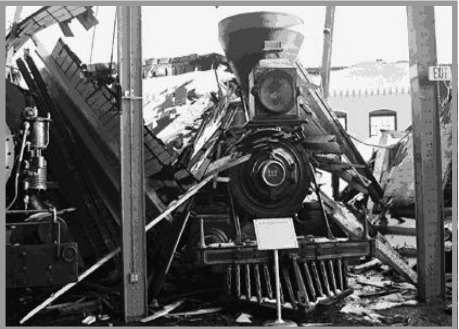
This is a portion of the damage to the B&O Museum in Baltimore done by the accumulation of an unusual amount of snow on the roof of the roundhouse and the subsequent collapse of a portion of the structure on Monday February 17. The above photo, from the B&O Museum website, shows some of the damage to the structure and B&O No. 117 "Thatcher Perkins," a ten wheeler locomotive.
